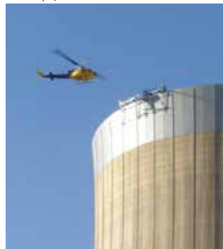
Chimney Repair, Tarong Power Station, QLD
