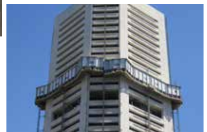
MLC Centre Facade Maintenance, NSW
