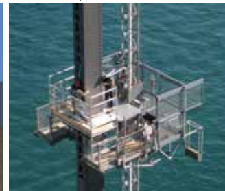
Sydney Harbour Bridge Maintenance, NSW
